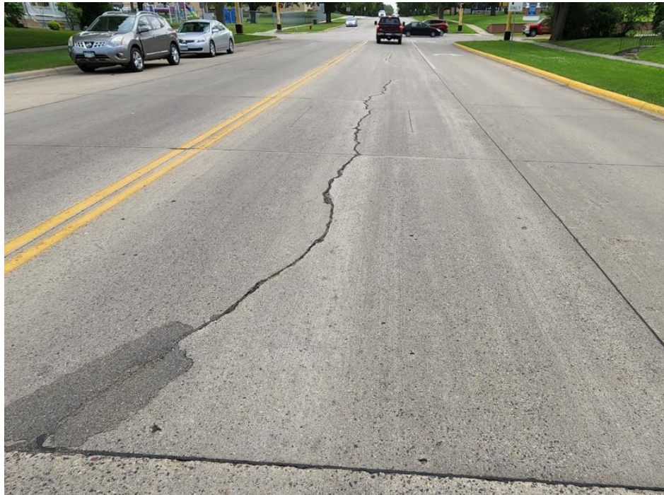
Figure 2-9 – Mid-Block between Lincoln Ave and Chambers Ave – Longitudinal Cracking
