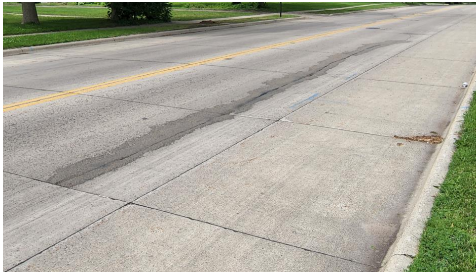
Figure 2-9 – Mid-Block between Lincoln Ave and Chambers Ave – Longitudinal Cracking
