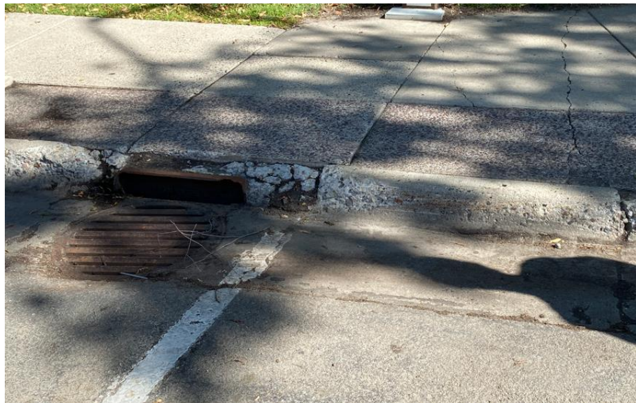
Figure 2-6 – In front of Central Park – Catch basin with deterioration.
