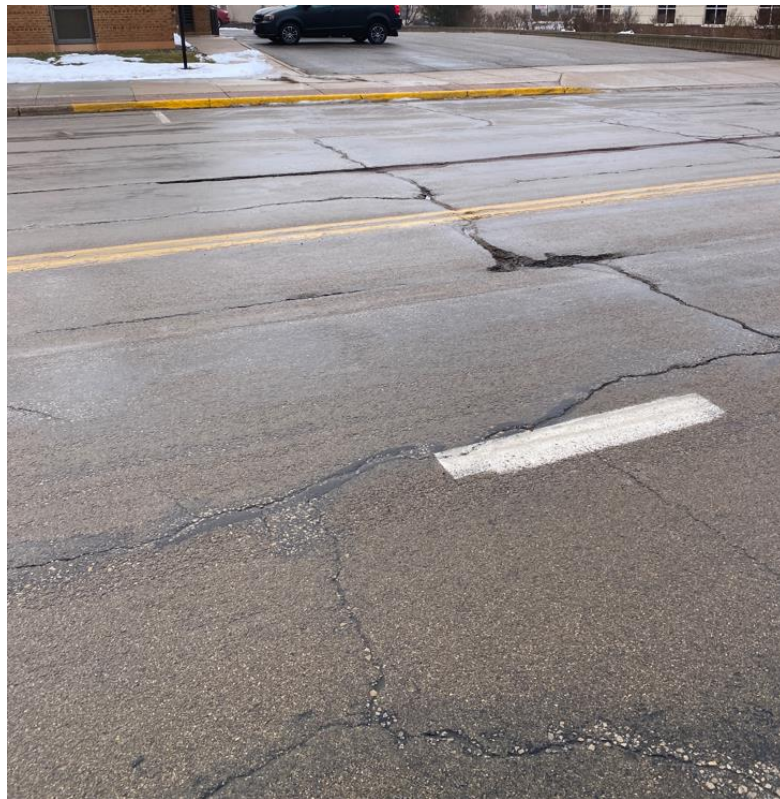
Figure 2-2 – East of Oak Ave and Main St Intersection – Shows cracking, resulting in potholes.
