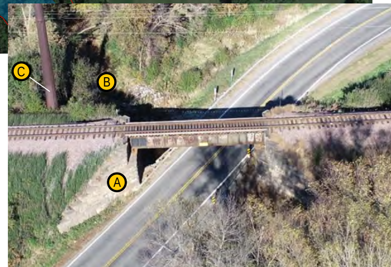
UAS Photo of Existing RR Bridge
