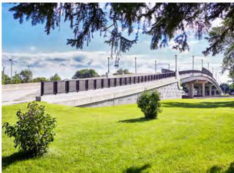
12th Street NW UPRR Overpass
