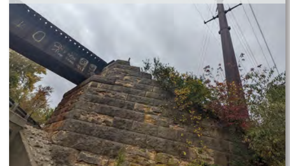
SMMPA Overhead Transmission Tower in NW Quadrant of Existing Bridge
