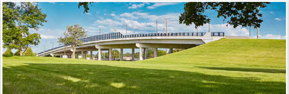
19th Street SW UPRR Overpass
