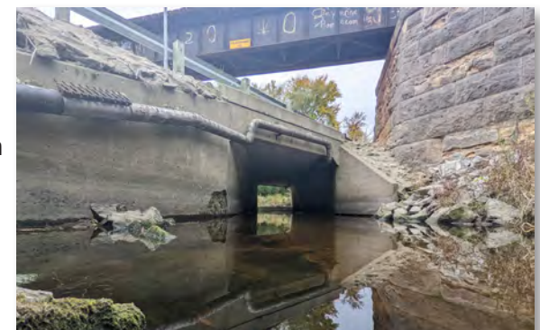
Existing box culvert beneath CR 180, looking downstream
