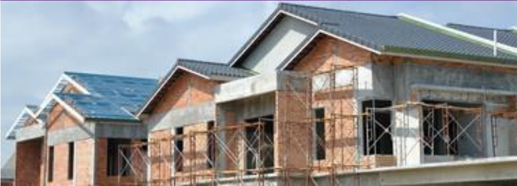
Housing Infrastructure Programs
